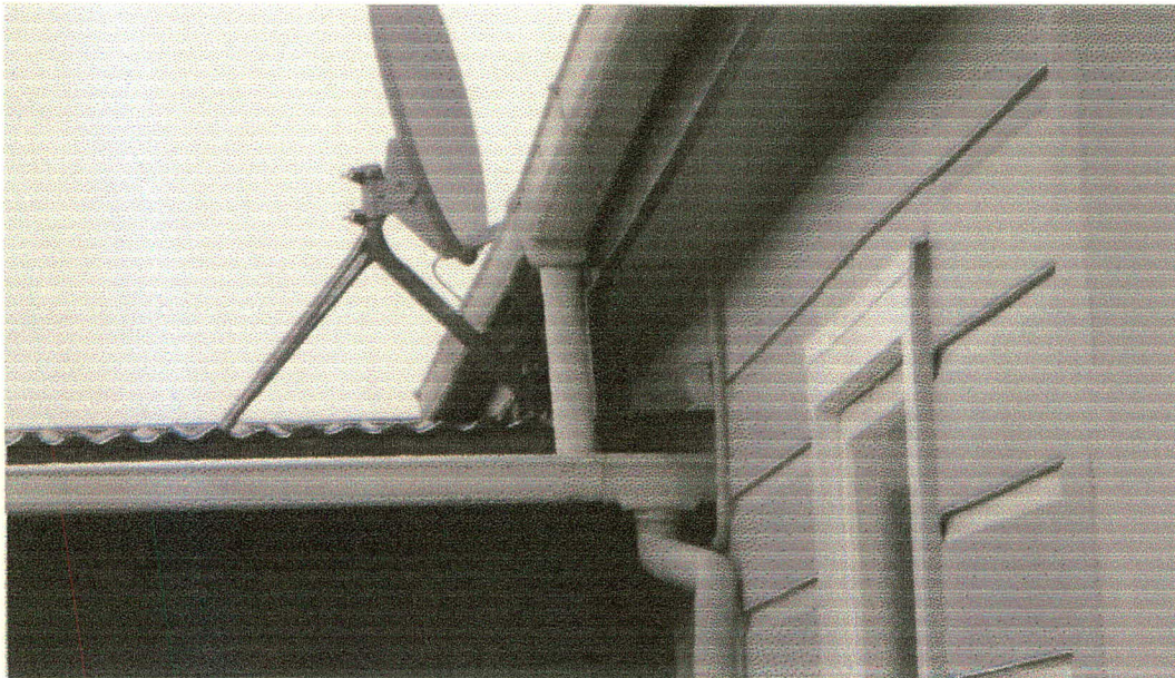
Kitchen roof to wall junction
