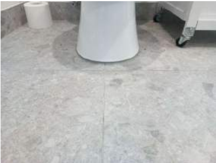
Toilet sealed to the floor
