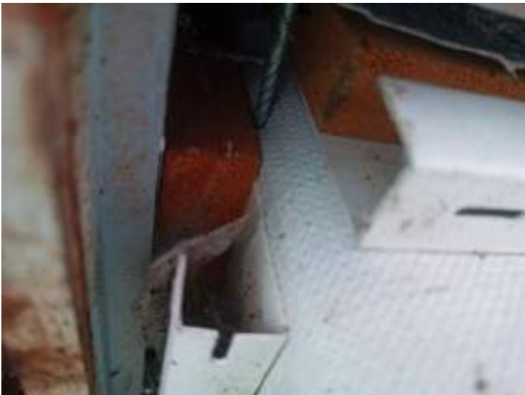
Vented cavity and building wrap visible
