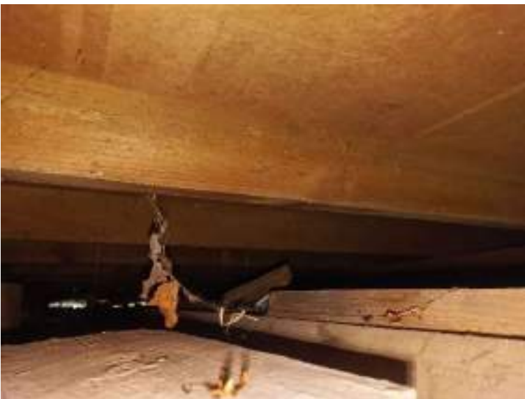
Original flooring and floor framing below the sleepout
