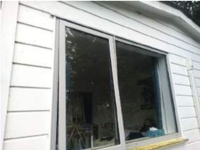
All flashings to windows and doors appear to be installed correctly
