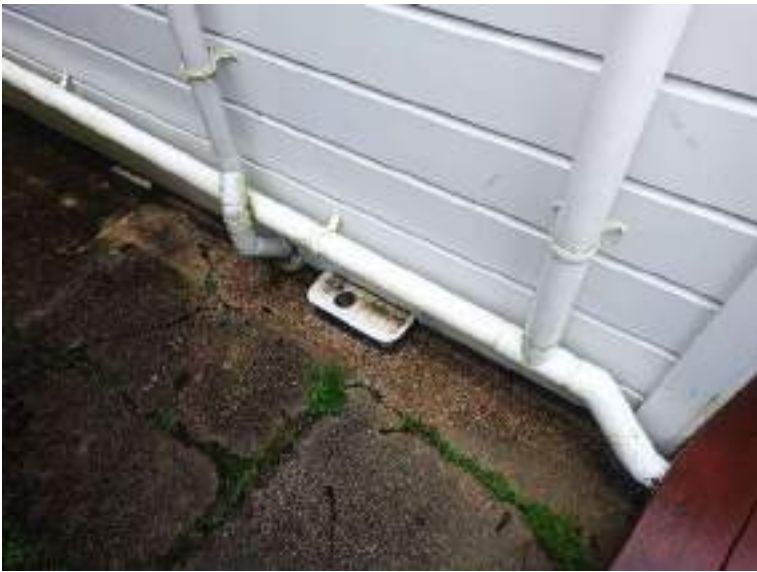
Gully trap and plumbing outside the ensuite
