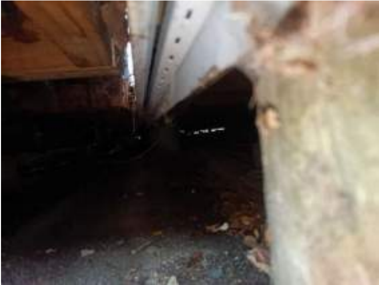
Vented cavity visible
