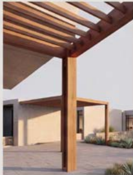
Timber Work & Concrete Coexistence
