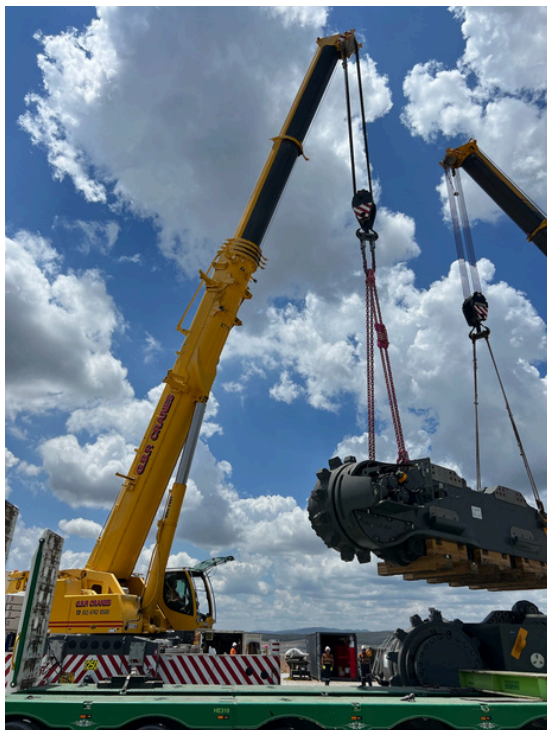
Dean-0 Sling assisting in lifting an undercarriage of an excavator
