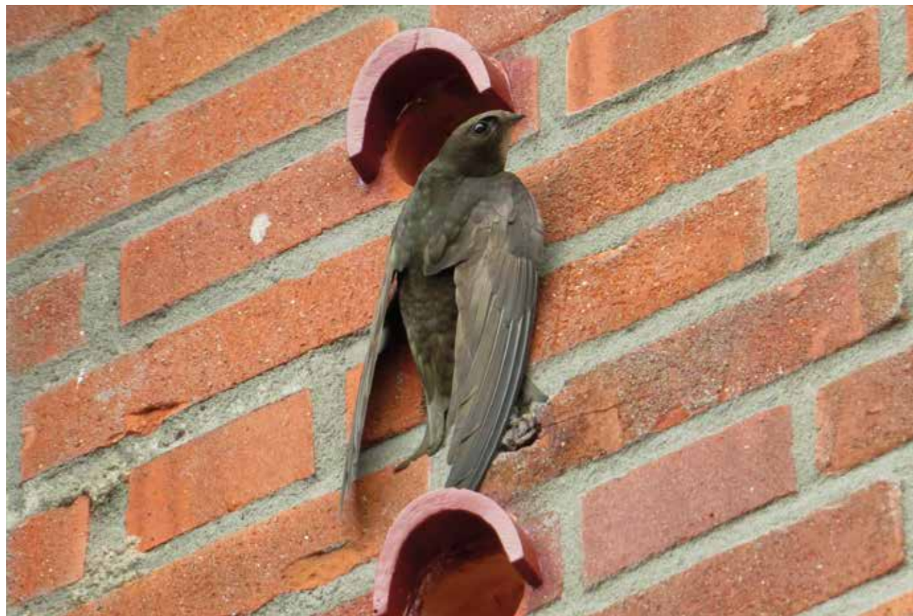
▲ A swift using swift bricks, which are hollow and contain internal nest boxes. © XJochemx.nl | CC-BY-SA 4.0
