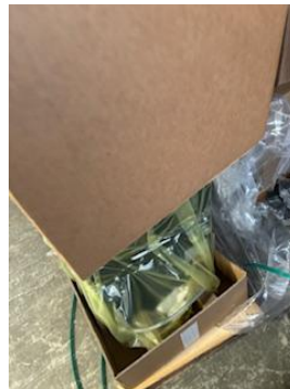
Step 2: Removing compressor box
