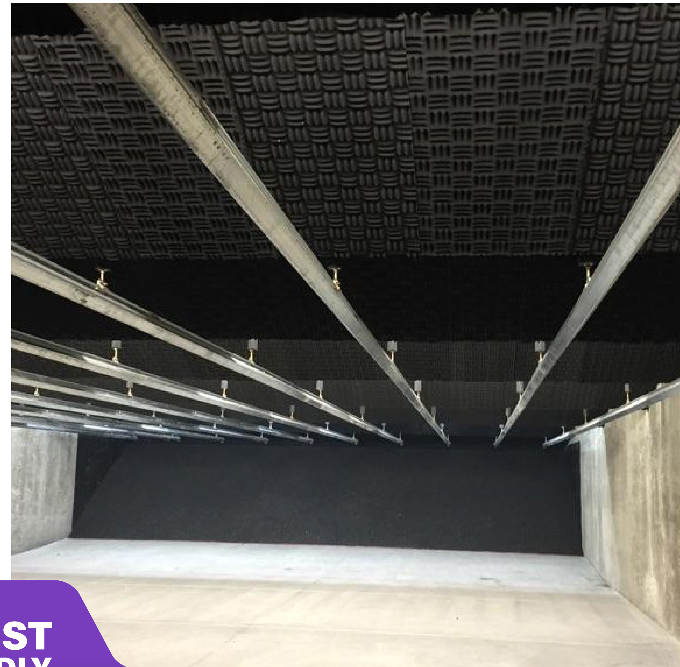
Baffles prevent noise transmission
