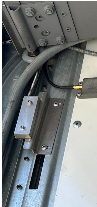
Figure 49 Door Sensor mounting Roll up Door
