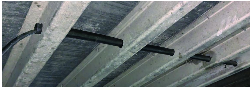
Figure 31 Wire Routing Example
