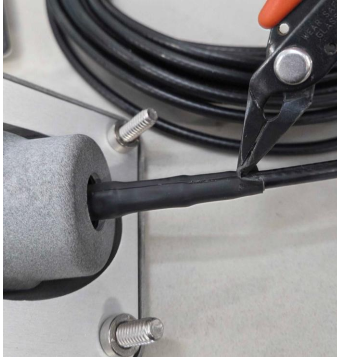
Figure 38 Use pliers to grip the cut edge and begin peeling the sleeve
