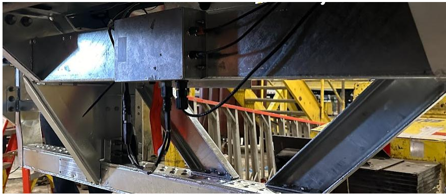
Figure 6 Example of camera enclosure near door frame
