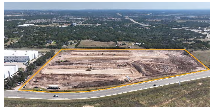
Project Completion: Ready for Tenant Occupancy
