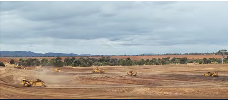
Earthworks during construction of the water storage for the unleased portion of Rookwood Farms, central Queensland, May 2026.
