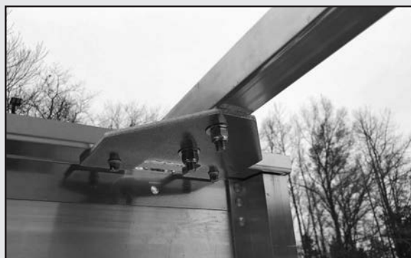
View of cross bar from underside bracket, showing two bolts per side
