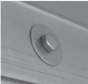
Close up of bolt through washer and mounting angle
