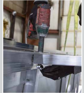
Below Cross Bar View
