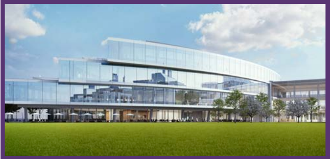
Exterior of Expedia Group Seattle HQ Building
