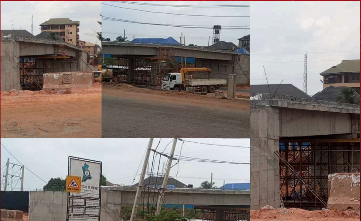
THE AWKA FLYOVER STILL UNDER CONSTRUCTION advokc
