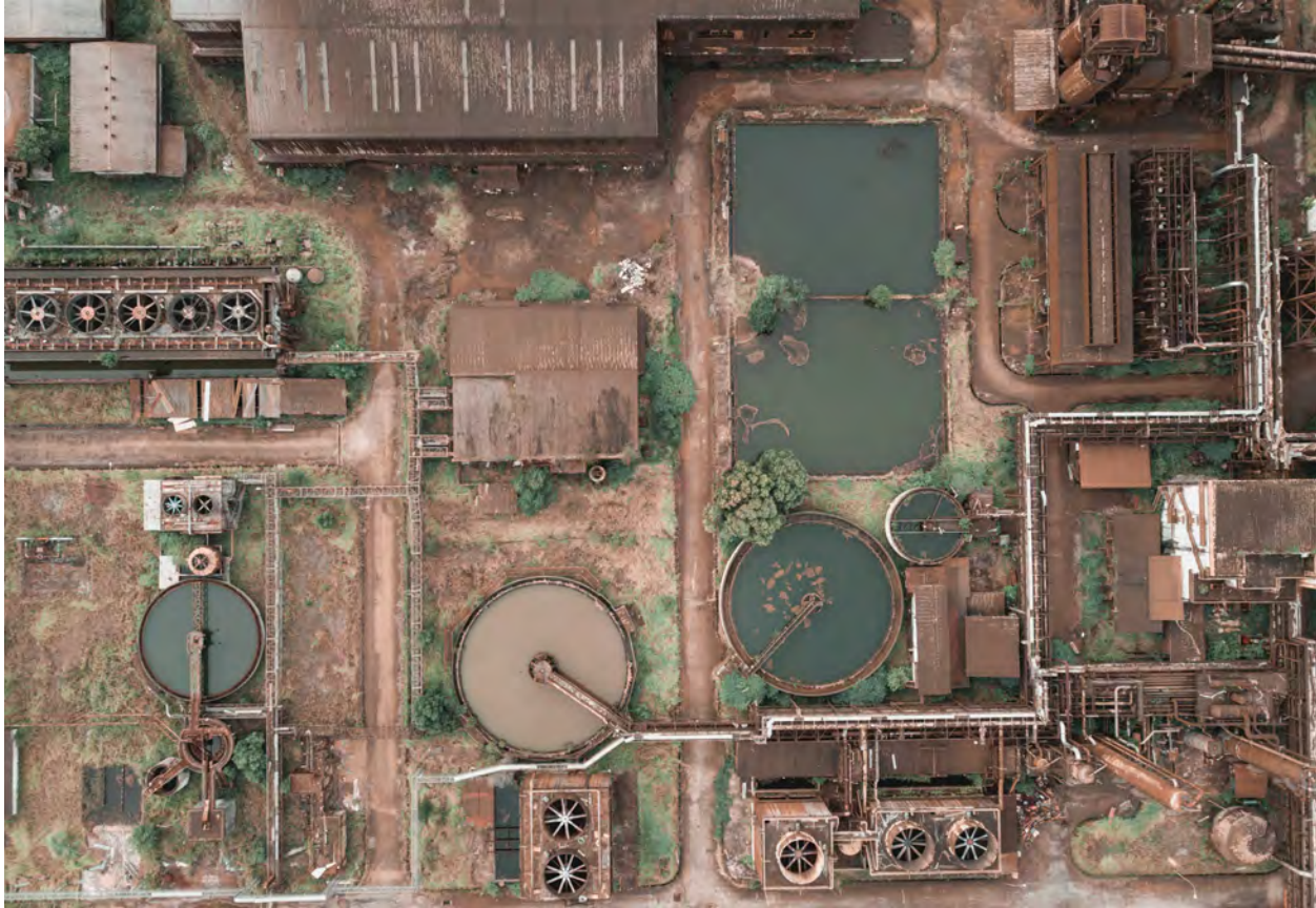
Purification tanks of old wastewater treatment plant © Pok Rie_Pexels
