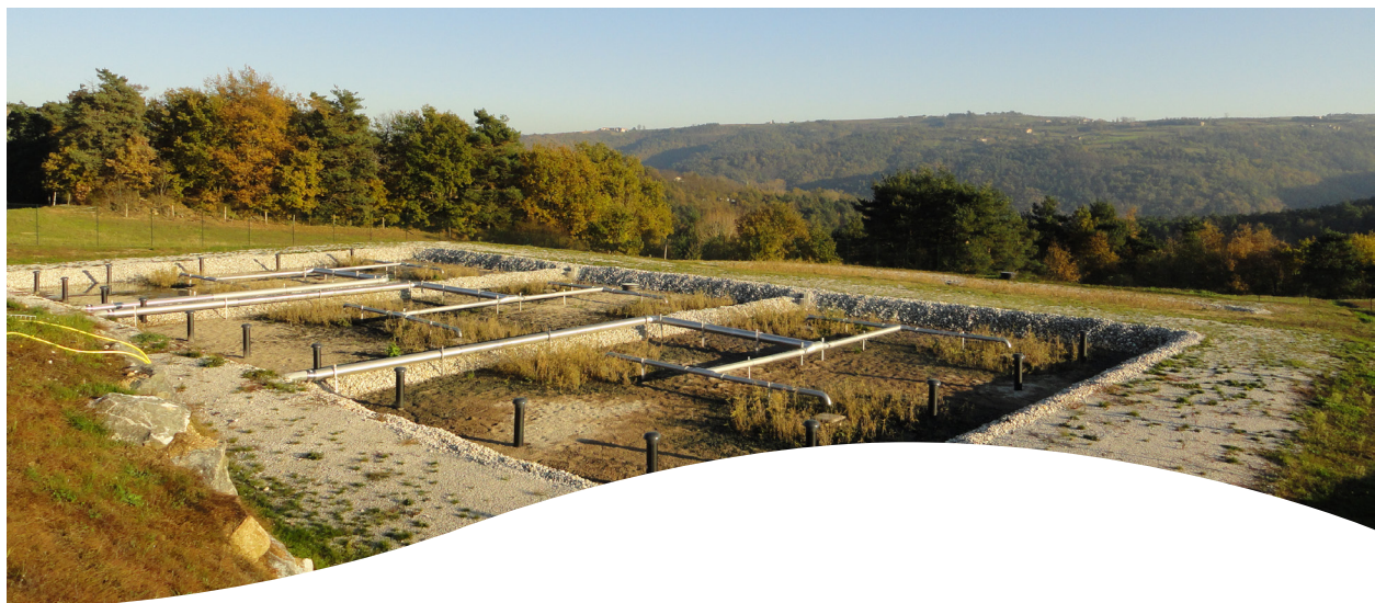
Vertical Flow Constructed Wetland with Sludge Mineralisation © Florian Klingel and Pierre-Henri Dodane Flickr CC BY 2.0
