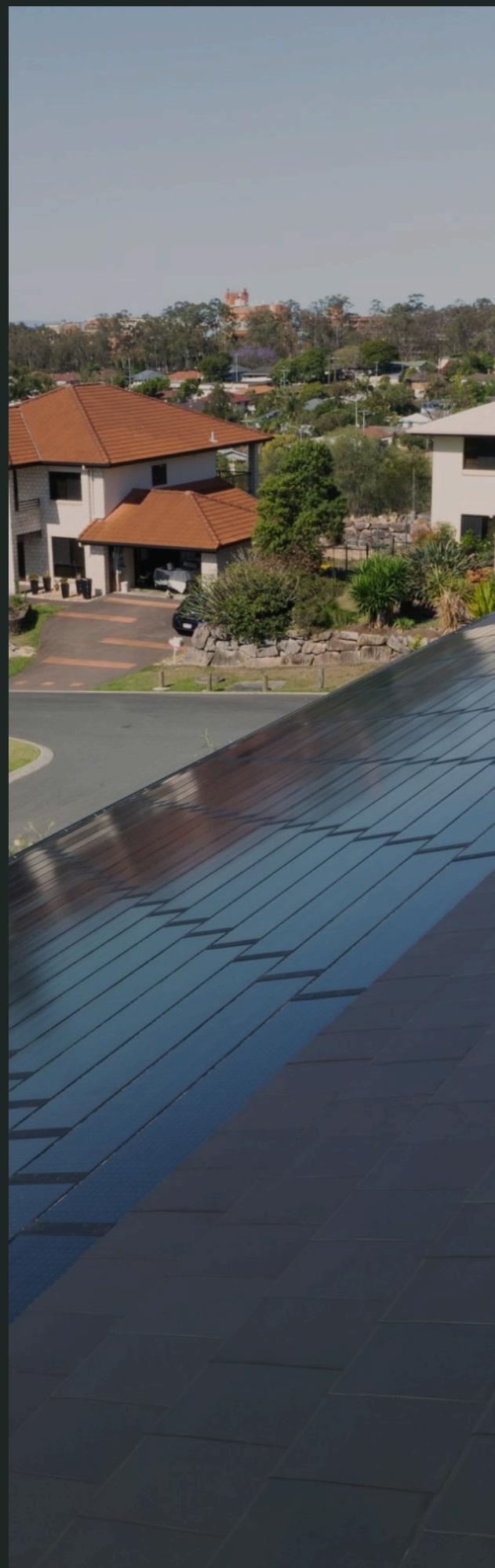
The upgrade was delivered as a coordinated roofing and solar project, with close collaboration between Bristile Roofing's contractors, Solar Install Co (a Volt Installation Partner), and Volt's technical team, who provided direct onsite support throughout the installation. Sections of the roof were stripped back, new sarking and battens installed for the new solar tile system.
