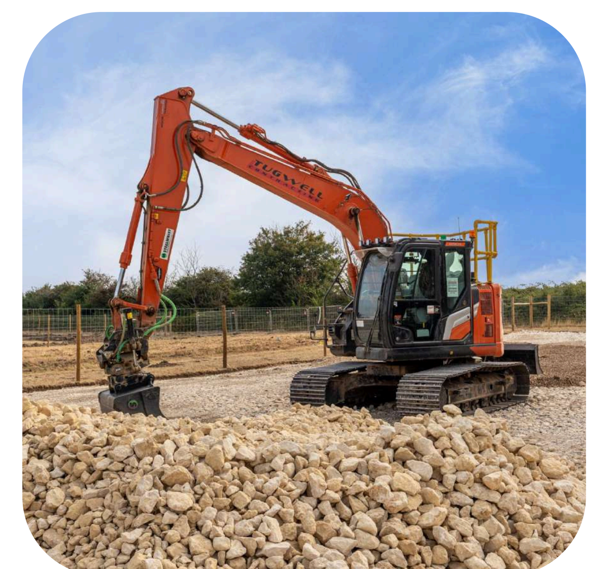
Crushed stone access tracks & underground cables
