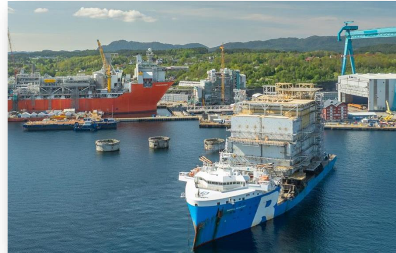
Foto: Aker Solutions, Stord Yard
