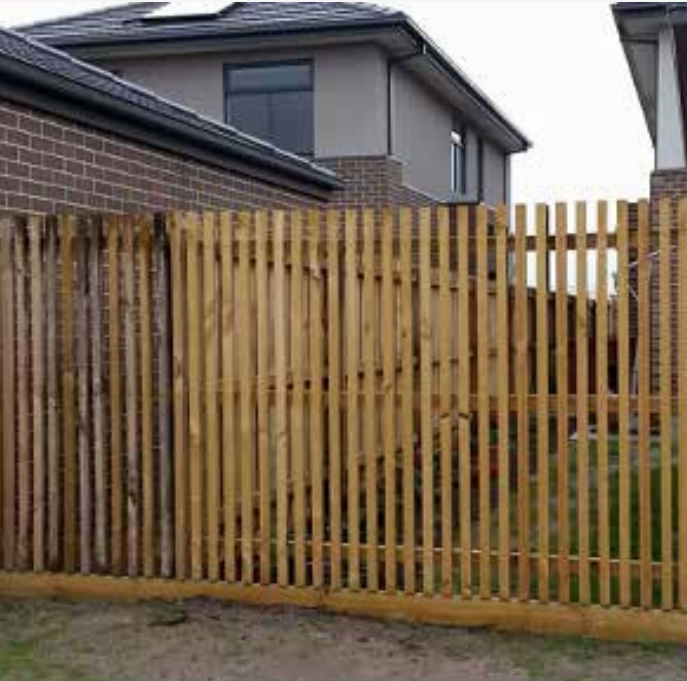
Rear Fence construction abutting a Public Open Space Reserve (if applicable):
