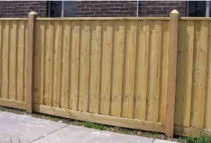
Standard Rear Fence construction:
