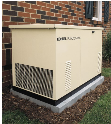
Standby generators are permanently wired into the home's electrical system by a qualified electrician. Photo credit: Kohler
