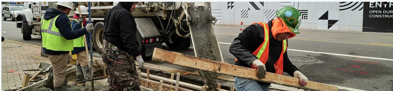
A concrete crew at work in Crystal City, Virginia, 2019. Carol M. Highsmith Archive, Library of Congress.
