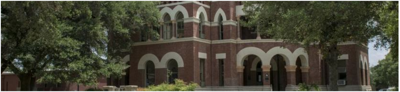
The Gonzales County courthouse, Gonzales, Texas, 2014. Carol M. Highsmith Archive, Library of Congress.
