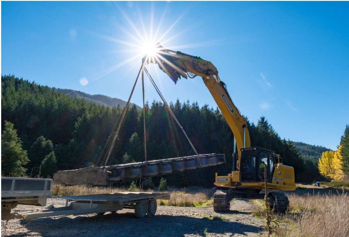
Bridge installation at Renwick Forest (Ernslaw One)
