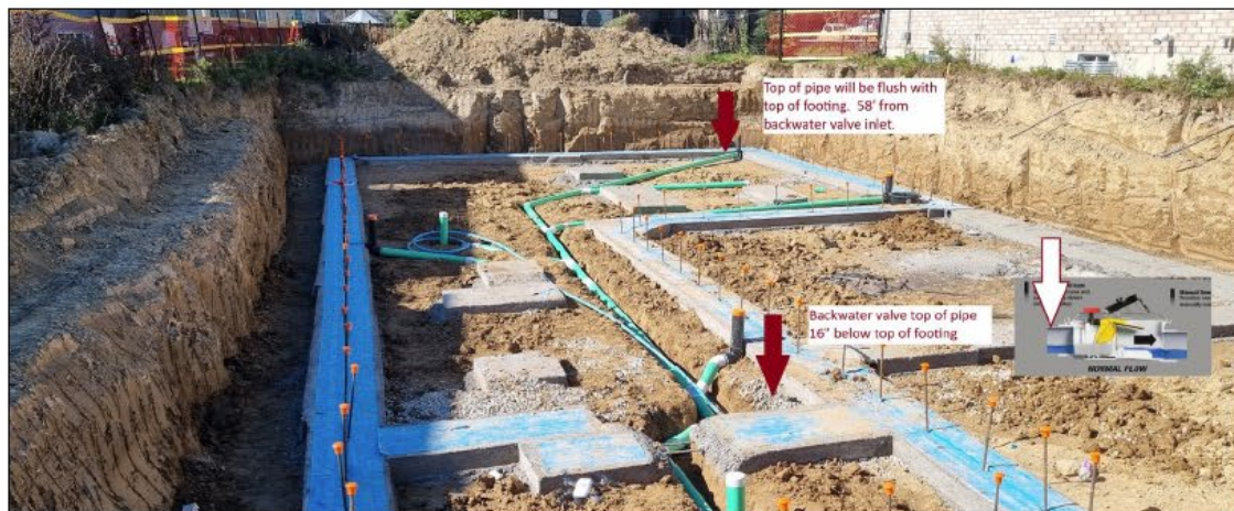
Building Drain, Sewer Slope, run (Nov. 2025)
