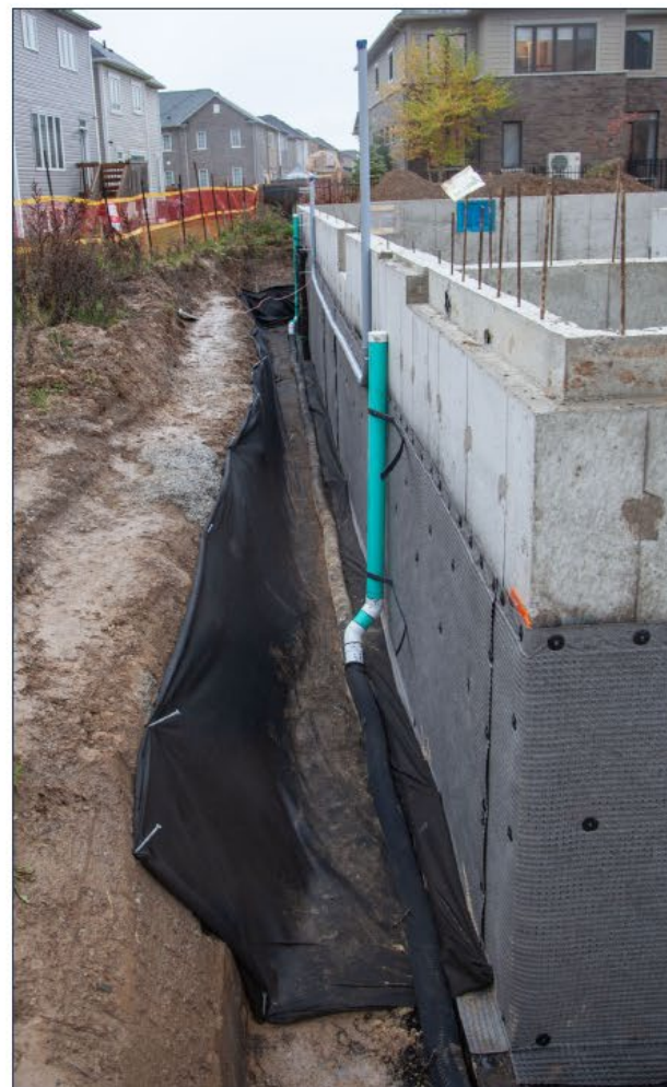
Foundation drain access (Dec. 2025)
