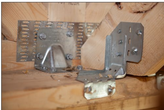
Gable End Wall Bracing (Jan. 2026)
