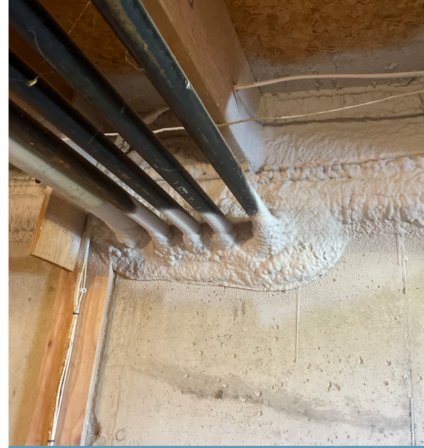
Above: Finding and addressing the major sources of air leakage take priority. Basement headers are a common example.
