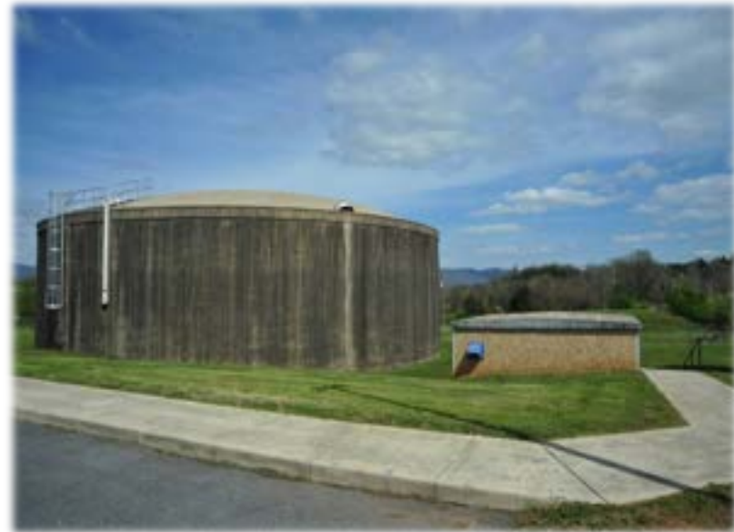
Photo WTP Staff, Finished Water Tank – 2 Million Gallons
