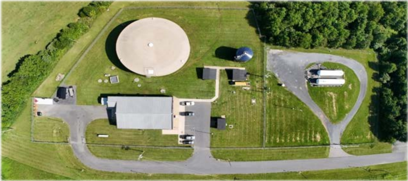
Photo Ben Glenn, Water Treatment Plant Stoney Brook Lane
