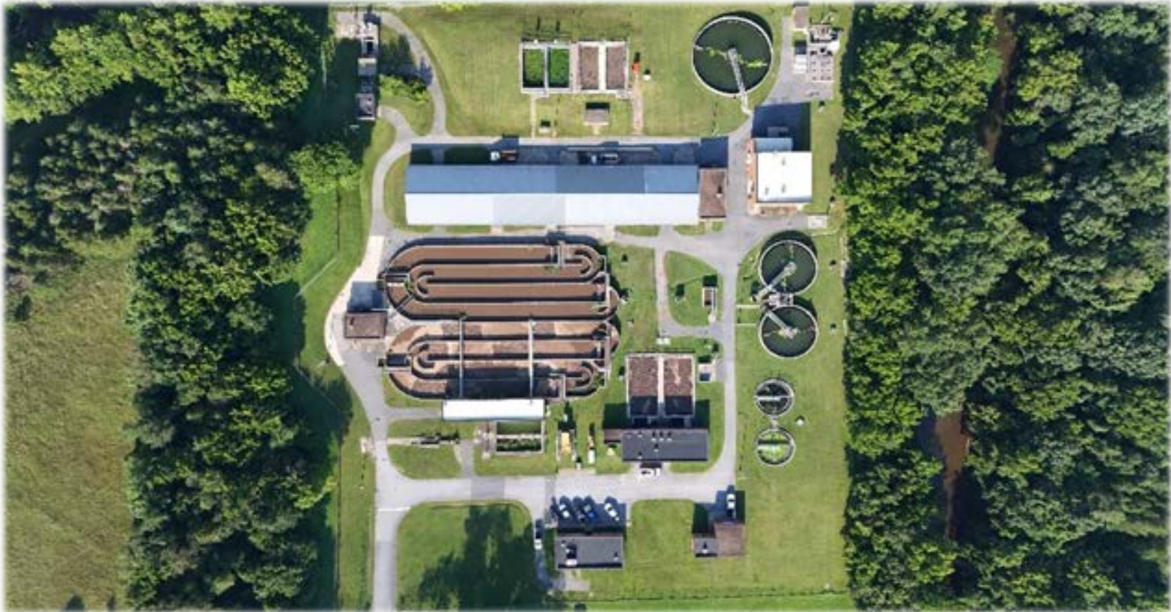
Photo Ben Glenn, Waste Water Treatment Plant After its 2010 upgrades to meet the Chesapeake Bay effluent quality standards
