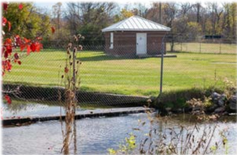
Photo Town Staff - Hite Spring Pump House
