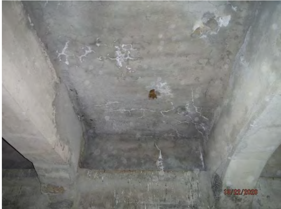
SPAN 3, BAY 2 DECK UNDERSIDE. NOTE MOISTURE SEEPAGE AND EFFLORESCENCE.
