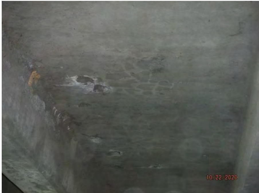
SPAN 4, BAY 2. NOTE MOISTURE SEEPAGE.
