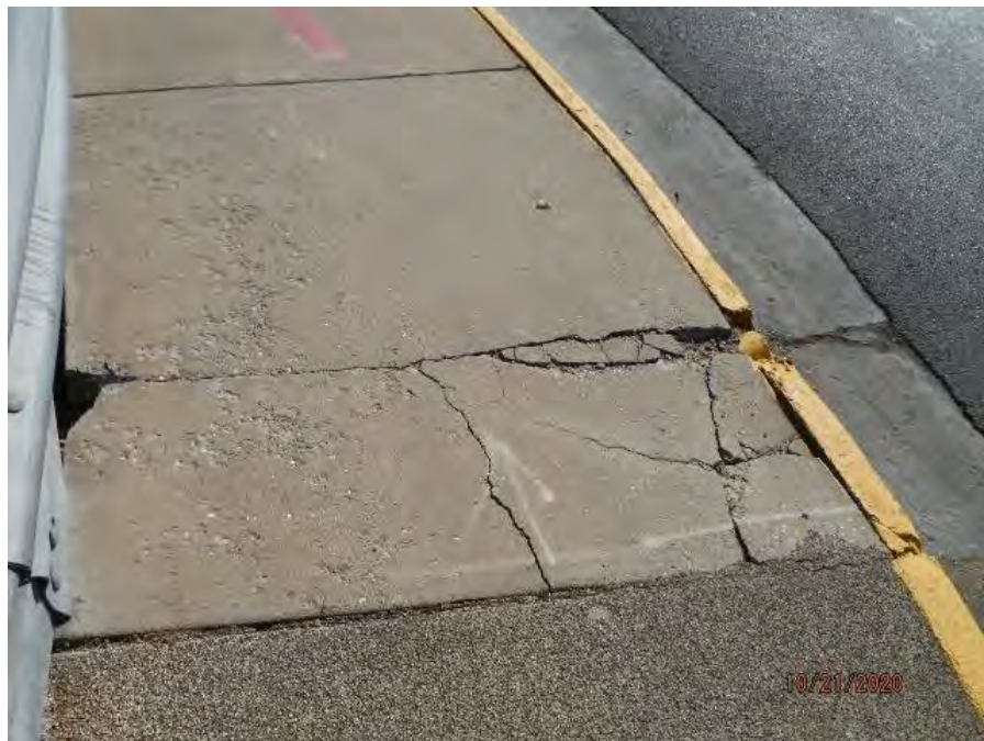
DOWNSTREAM APPROACH SIDEWALK AT BARREL #6 CRACKED/BROKEN FOR 25 SF.
