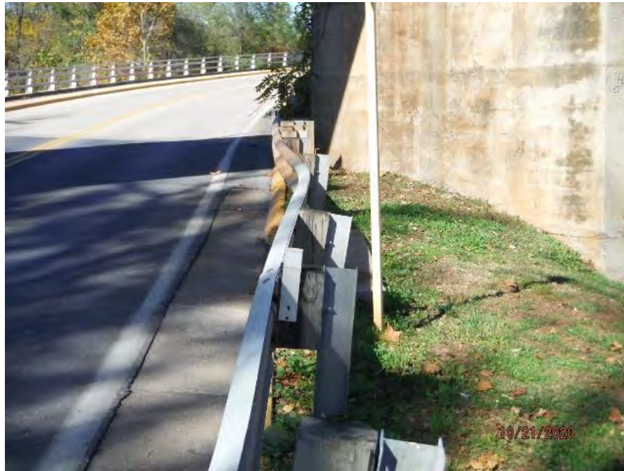
ABUTMENT A UPSTREAM GUARDRAIL. NOTE IMPACT DAMAGE.
