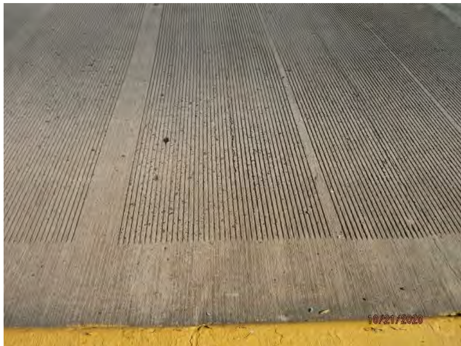
SPAN 2 DECK, DOWNSTREAM LANE. NOTE CRACKING.
