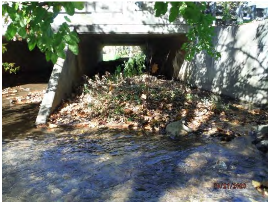
STREAMBED AGGRADATION IN BARREL #6.
