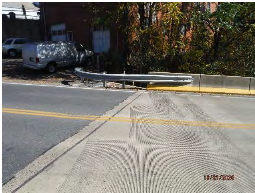
ABUTMENT B UPSTREAM GUARDRAIL. NOTE NONSTANDARD GUARDRAIL.
