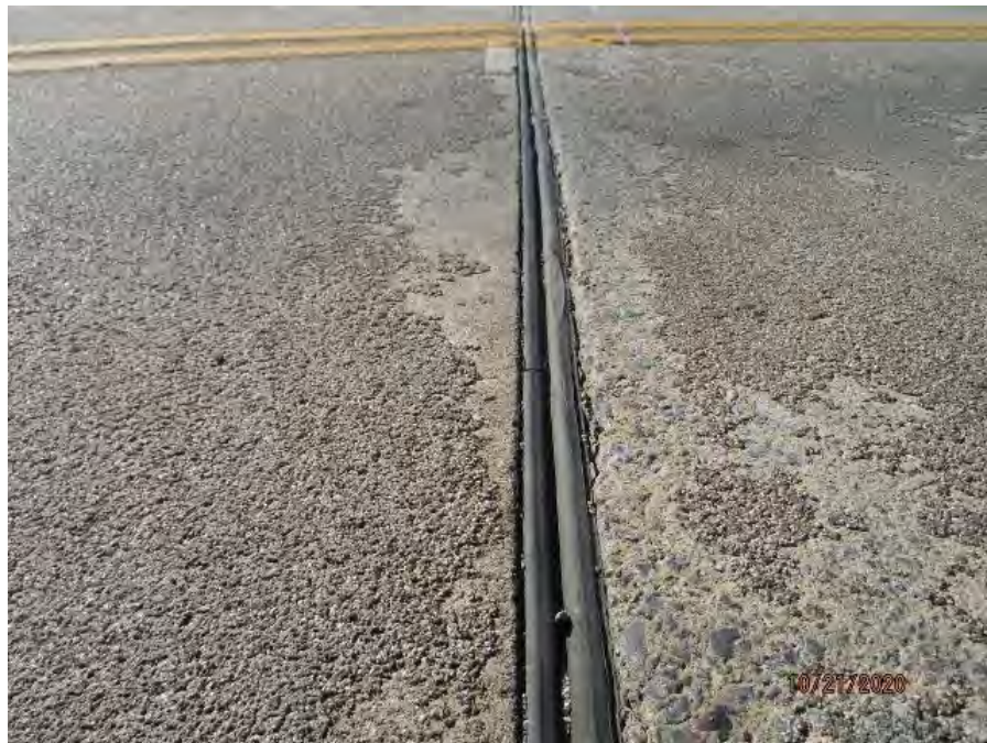
ABUTMENT B JOINT LEAKING.
