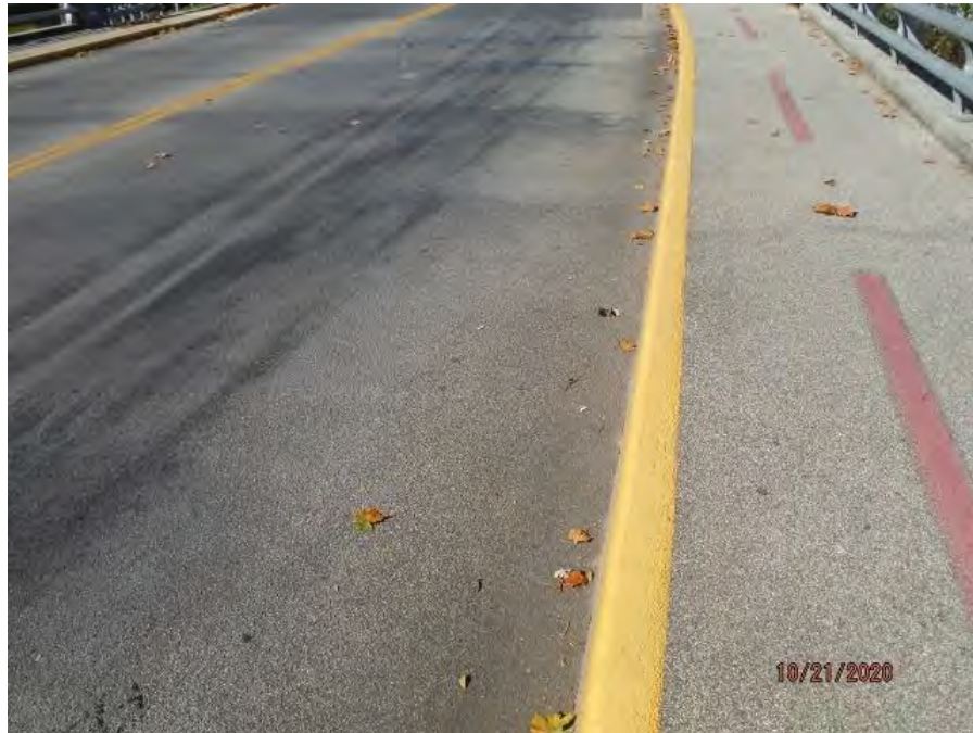
TOP OF DECK AND SIDEWALK. NOTE SAND/EPOXY OVERLAY.
