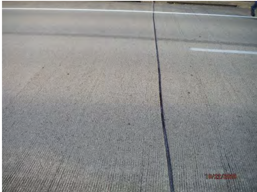
PIER 4 JOINT LEAKING.
