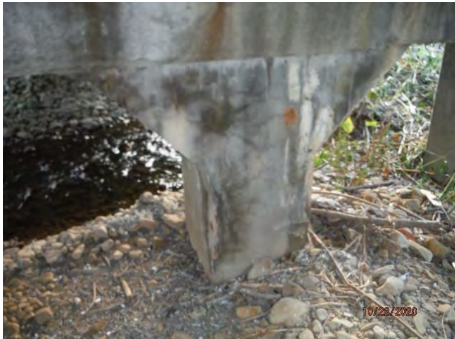
PIER 3, COLUMN 3. NOTE DELAMINATED CONCRETE.
