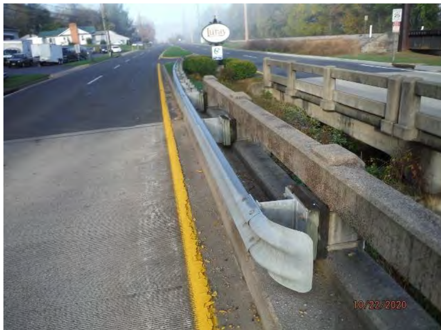
ABUTMENT A APPROACH GUARDRAIL, LEFT SIDE.
