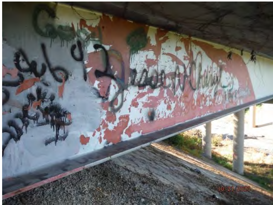
ABUTMENT A, BEAM 5 PAINT CONDITION.
