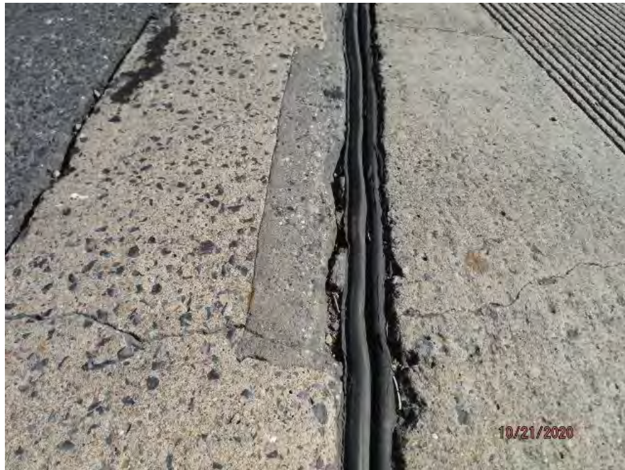
ABUTMENT B JOINT. NOTE COMPRESSION JOINT SEAL LEAKING.
