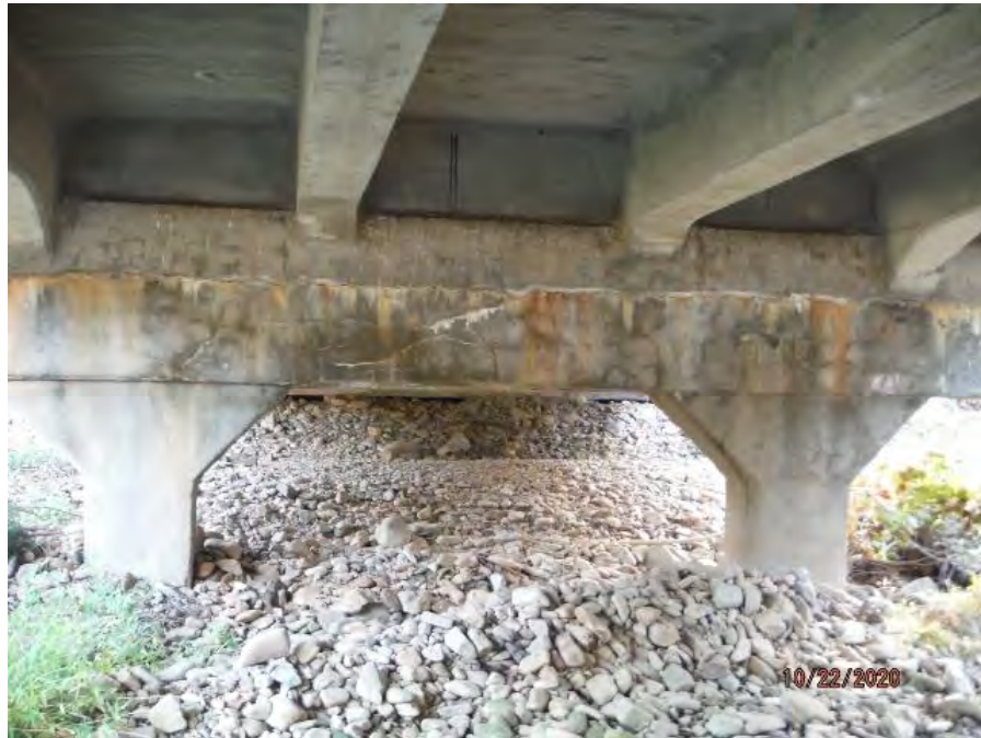
PIER 4 CAP. NOTE DELAMINATED CONCRETE WITH EFFLORESCENCE.
