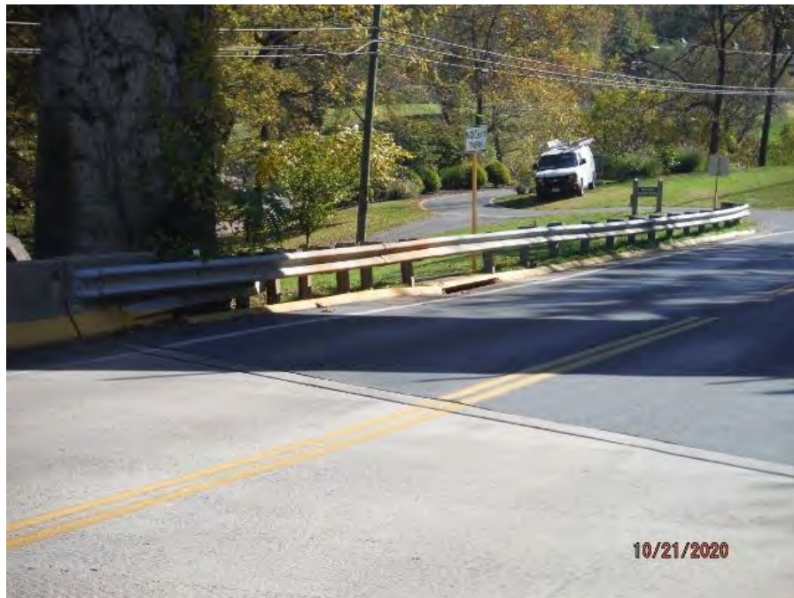
ABUTMENT A UPSTREAM GUARDRAIL. NOTE NONSTANDARD GUARDRAIL.
