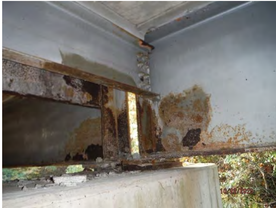
PIER 1, BEAM 5. NOTE PAINT FAILURE.
