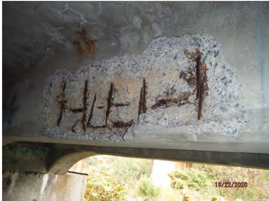
SPAN 5, BEAM 2. NOTE SPALLED CONCRETE.
