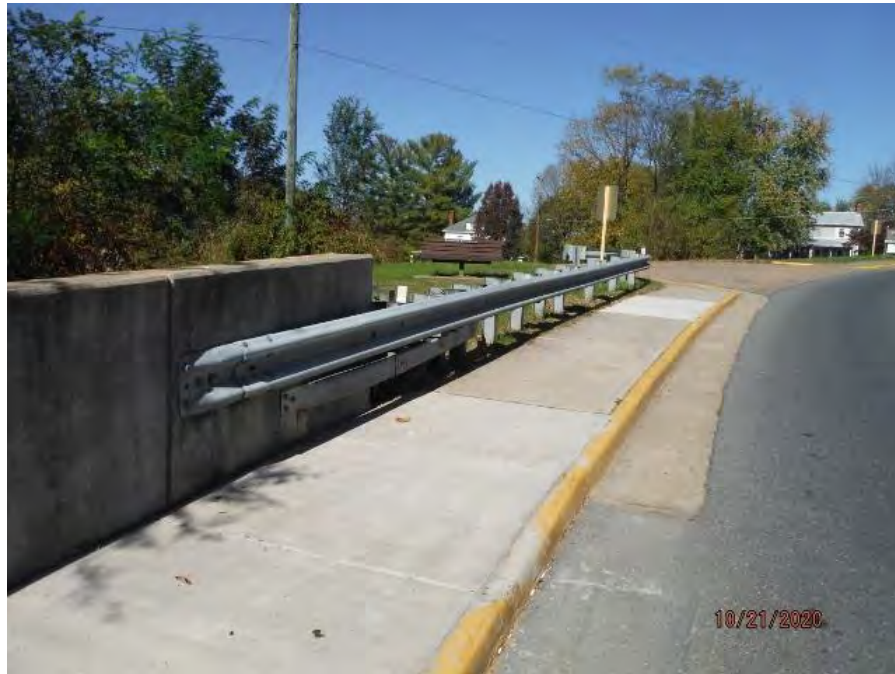
ABUTMENT B DOWNSTREAM GUARDRAIL. NOTE NONSTANDARD GUARDRAIL.
