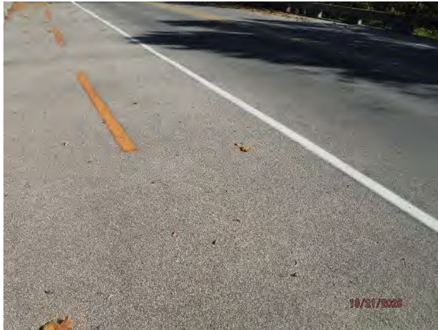
TOP OF DECK, DOWNSTREAM. NOTE SAND/EPOXY OVERLAY.
