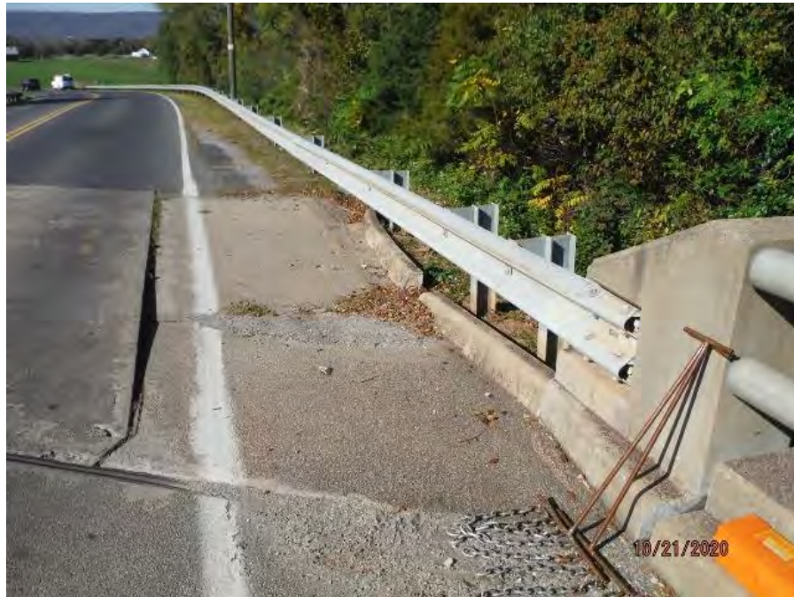
ABUTMENT B RIGHT SIDE APPROACH GUARDRAIL.
