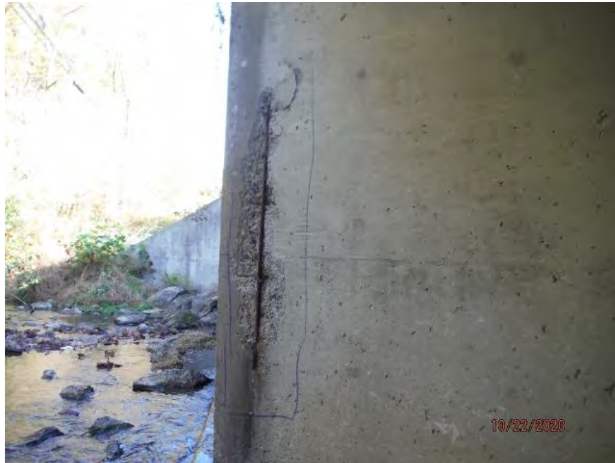
SPALL/DELAMINATION IN BARREL #1.
