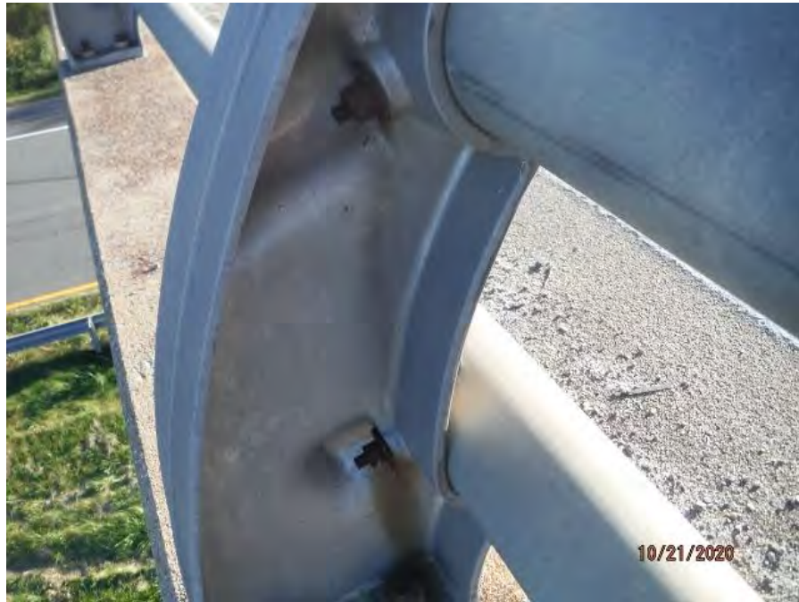
ALUMINUM RAIL. NOTE DISSIMILAR METALS REACTION.
