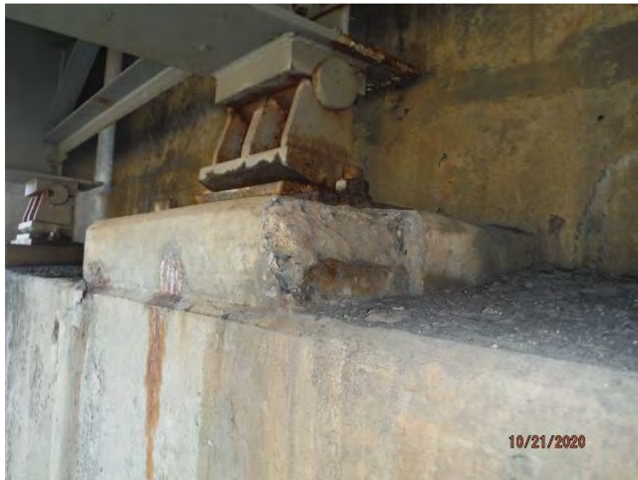
ABUTMENT A, BEAM 4. NOTE BEARING SEAT SPALL.
