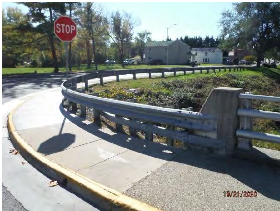
UPSTREAM APPROACH GUARDRAIL AT BARREL #6.
