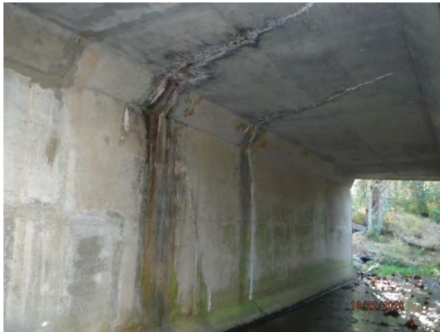
LEAKING CRACK IN BARREL #4 DOWNSTREAM END.
