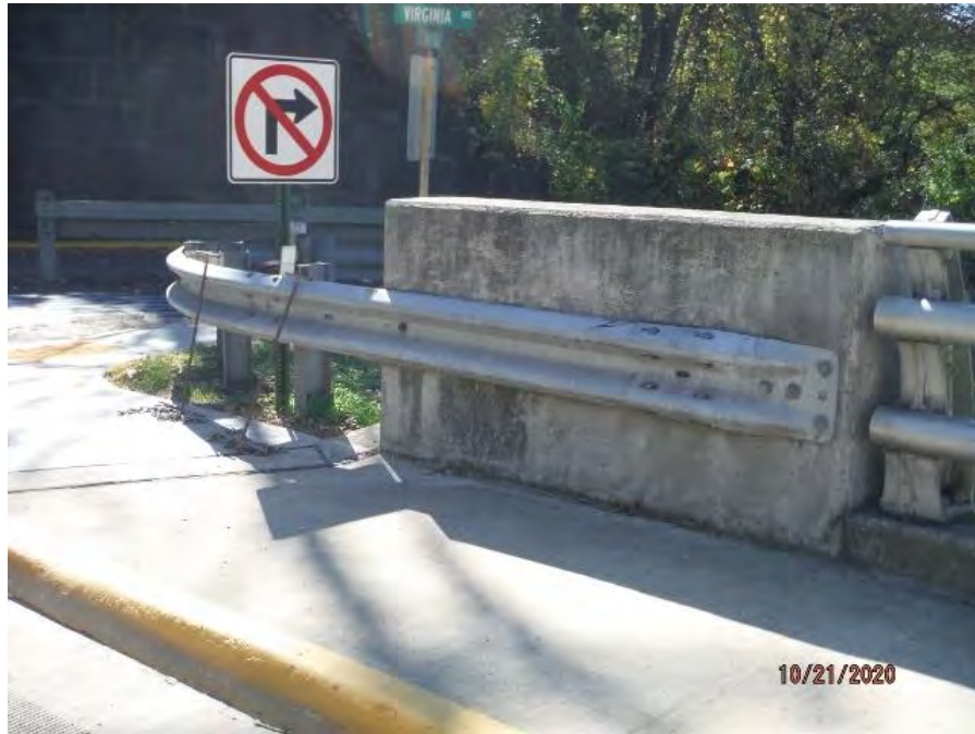
ABUTMENT A DOWNSTREAM GUARDRAIL. NOTE NONSTANDARD GUARDRAIL.
