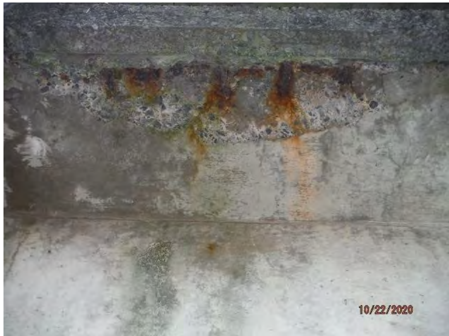
DECK OVERHANG, DOWNSTREAM SIDE. NOTE SPALLED AND DELAMINATED CONCRETE.
