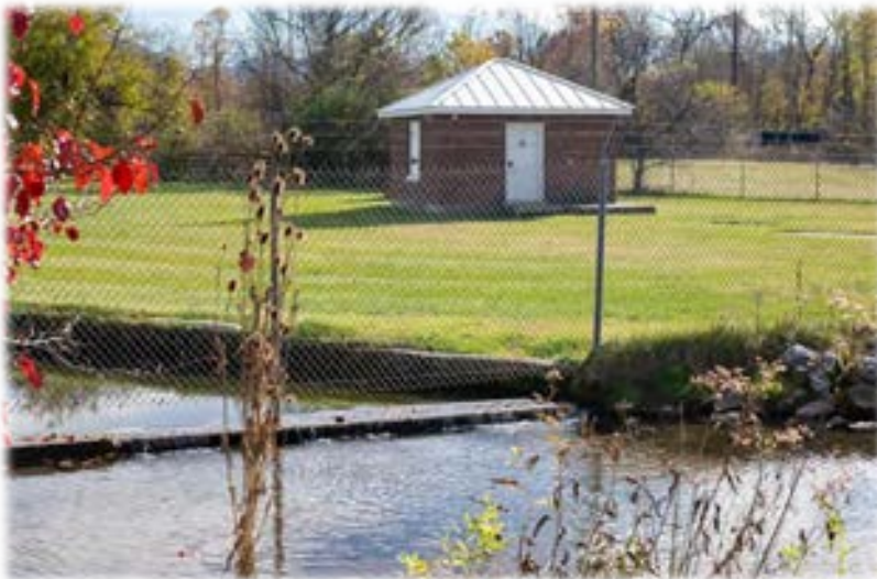
Photo Town Staff - Hite Spring Pump House
