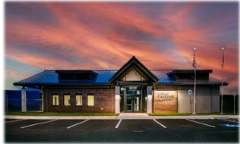
Photo Airport Website, Luray Caverns Airport Terminal
