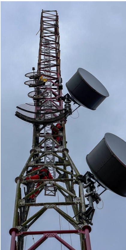
Access tower in place to remove top of the IT tower
