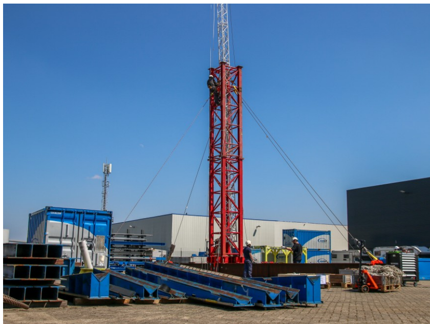
Testing the access tower at the Conbit yard
