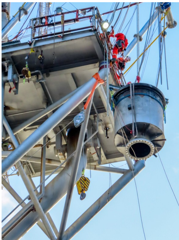
Flare tip hanging in flare tip handling system
