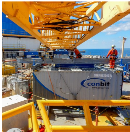
Crane boom on skidding system, supported by equipment container
