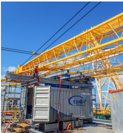
Crane boom on skidding system, supported by equipment container
