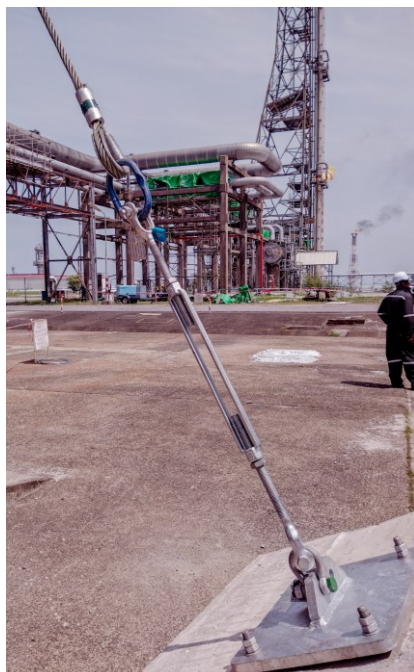
Tensioned guy wire secured to an anchor plate to stabilise the stack.
