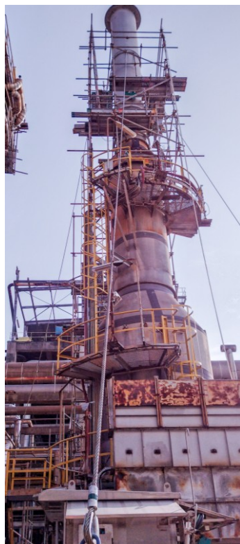
Crane and elevated platforms positioned around the stack for stabilisation work.
