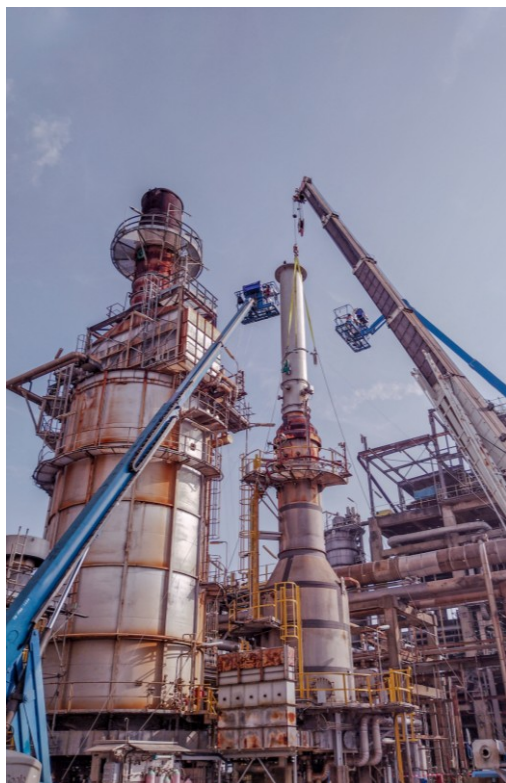
Crane and elevated platforms positioned around the stack for stabilisation work.
