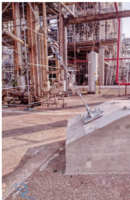
Tensioned guy wire secured to an anchor plate to stabilise the stack.
