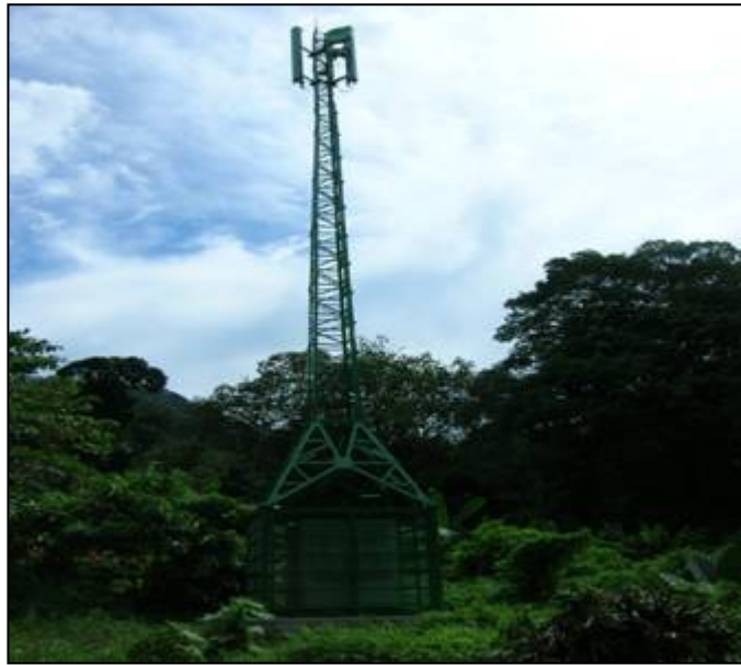
Rapid Mobile Structure
