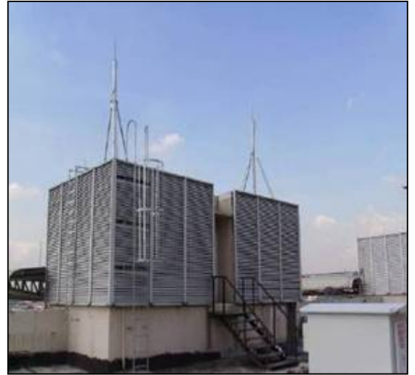
Standard Antenna & Microwave Pole / Tripod / Boom
