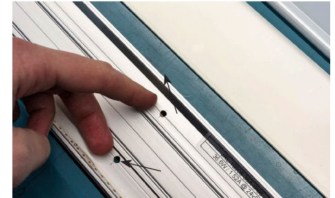
Step 4: Identify pre-drilled holes & use desired screws to mount the housing. (Drill additional screw holes as required along scribed line.)
