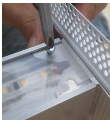
7A. Press the snap-fit lenses (wall section first) into the housings.
