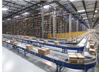
Integrated Conveyors and AS/RS
