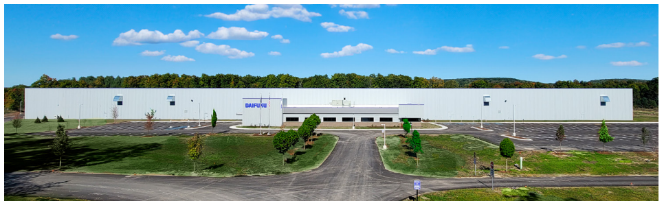
Northern Michigan Manufacturing Facility
