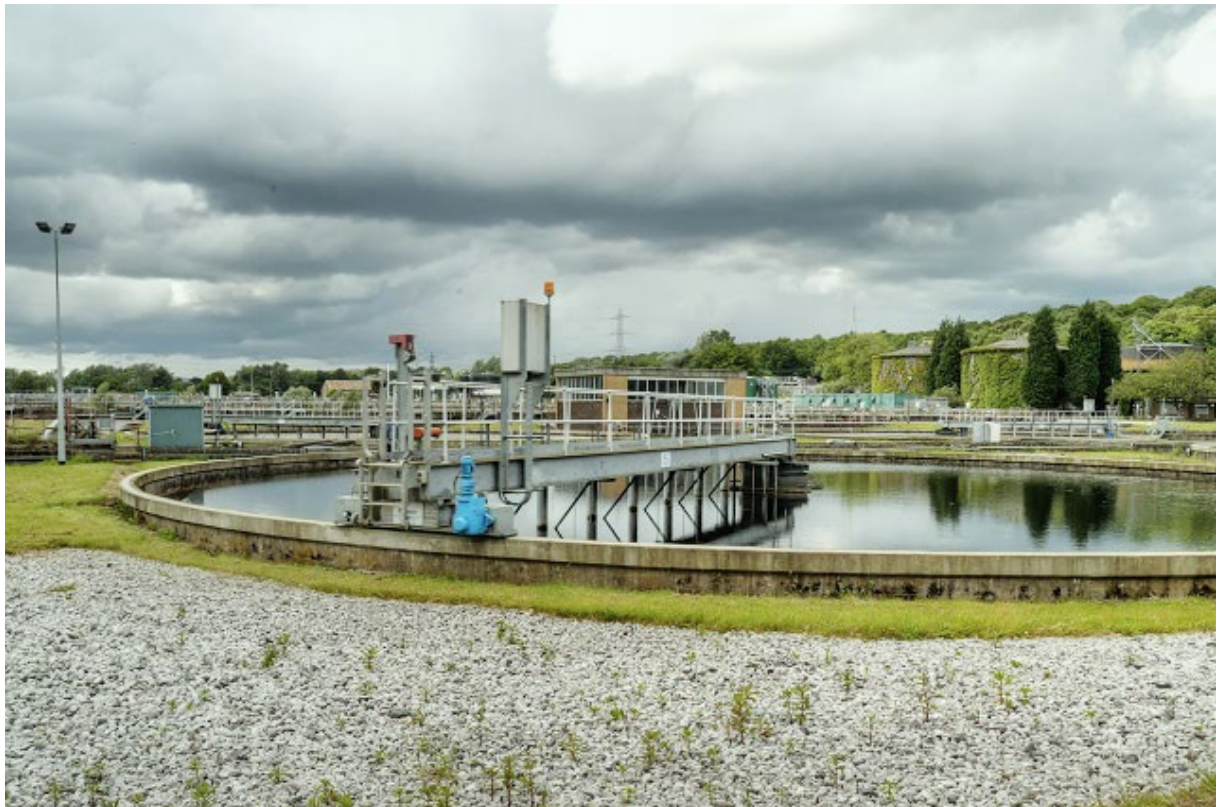
Figure 4: Sewage Treatment Plant
