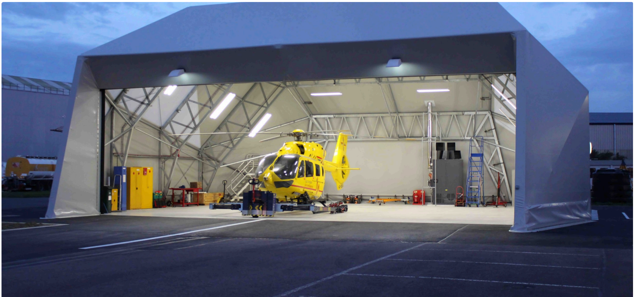
Fabspace V_02 hangar of the East Anglian Air Ambulance at Cambridge City Airport – produced in ten weeks, assembled in two. Photo: Fabspace Hangars GmbH
