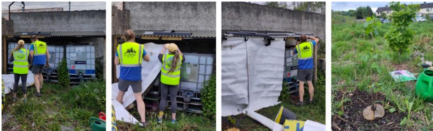
Adding a screen for the tanks based in McDonagh Crescent to protect them from sunlight, May 2025.
