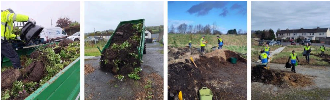
1 & 2) The Borough Council gives us waste plant matter, wood chippings & soil, Oct 2024. 3 & 4) We use it to level the site, Feb 2025.
