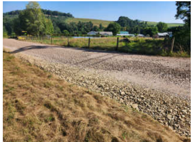
After - raised road and improved drainage
