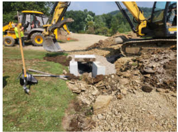
During - addition of drainage pipes
