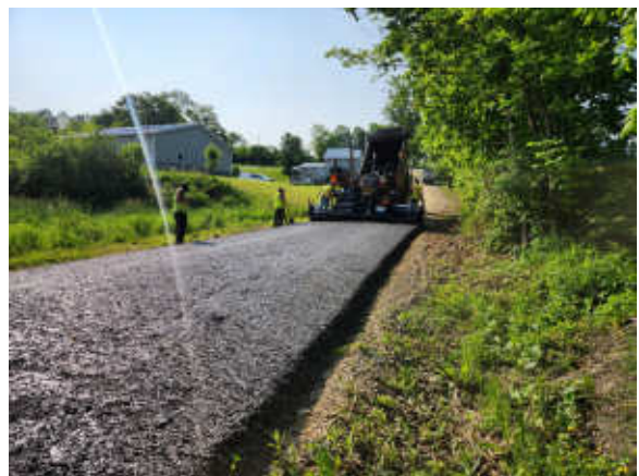
During - addition of fill
