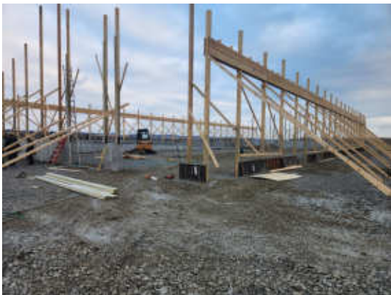
During - construction of framing
