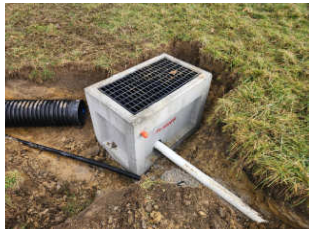
After - storm water outlet
