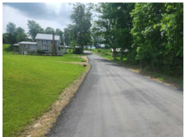
After - raised road and improved drainage
