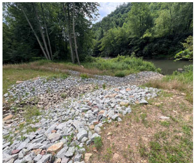
After - limestone outlet to Two Lick Creek
