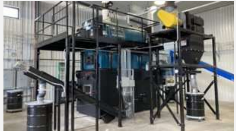
Fond du Lac Band of Lake Superior Chippewa Biomass District Heating System (Minnesota) installed a biomass district heating system for its Brookston Community Center, adding 3 MMBtu per hour of energy/ heating capacity. The system is projected to save approximately $31,000 annually. They celebrated with a ribbon cutting in June 2025. Photo by Josh Gregory / DOE
