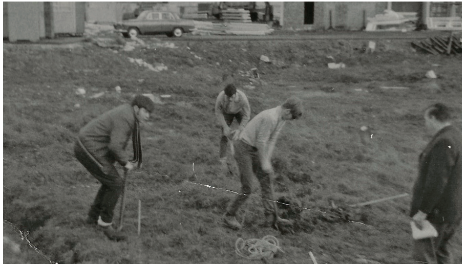
Wes (left) helping dig the foundations for Kingshurst Evangelical Church in 1971
