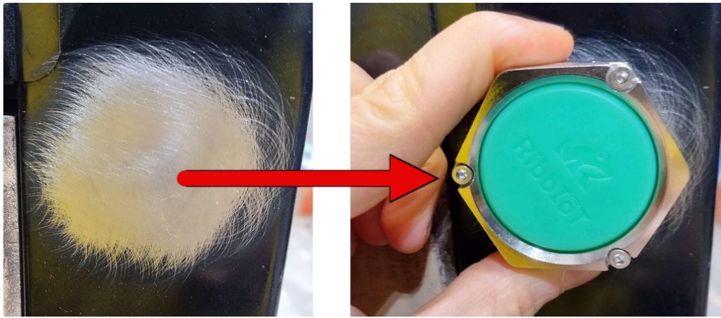
Paint removed locally (~2.5" diameter) prior to placing the Pod.
