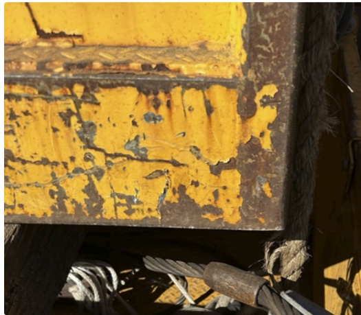
Painted surfaces that look like this must be ground prior to installation (remove all paint, rust, etc. locally where the Pod will be installed).
