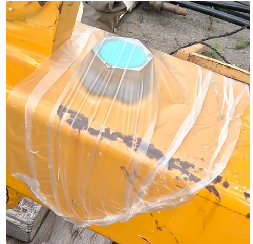
Step 6: If necessary, temporarily cover and protect the tracker from anticipated rain while the epoxy cures. This image shows GLAD PRESS'NSEAL applied.
