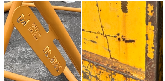
Step 1: Identify if necessary to grind away paint. The left image is an asset with brand new paint and OK to just clean IF appropriate. The right image represents an item where the paint must be removed prior to installation.
