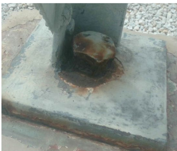
R27 Leg 4 - Kennedy Substation Base Plate/Anchor Nut Structural Condition: D
