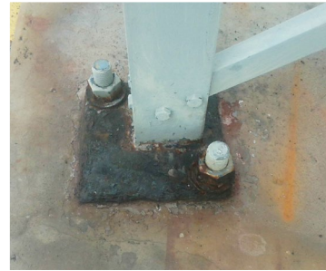
O12 Leg 1 - US1 Substation Base Plate Structural Condition: Priority
