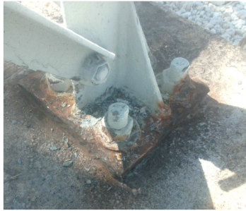
G6-1 Leg 2 - Stock Island Substation Base Plate Structural Condition: Priority
