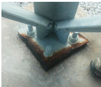
R27 Leg 4 - Kennedy Substation Base Plate Structural Condition: D
