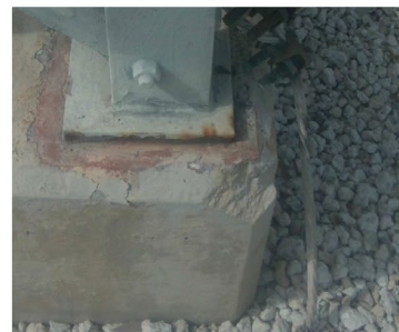
O16 Leg 3 - US1 Substation Concrete Foundation Condition: C
