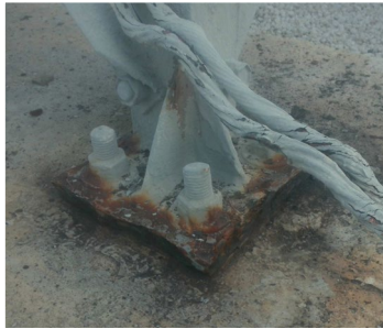
H8-1 Leg 2 - Stock Island Substation Base Plate Structural Condition: Priority
