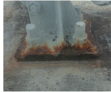
G8-1 Leg 2 - Stock Island Substation Base Plate Structural Condition: Priority
