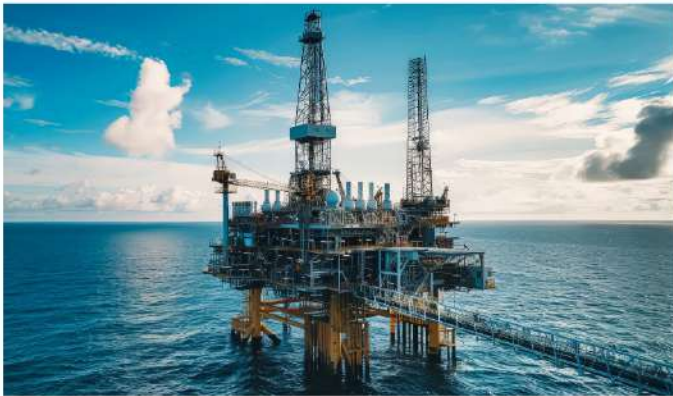
Rigs Onshore & Offshore
