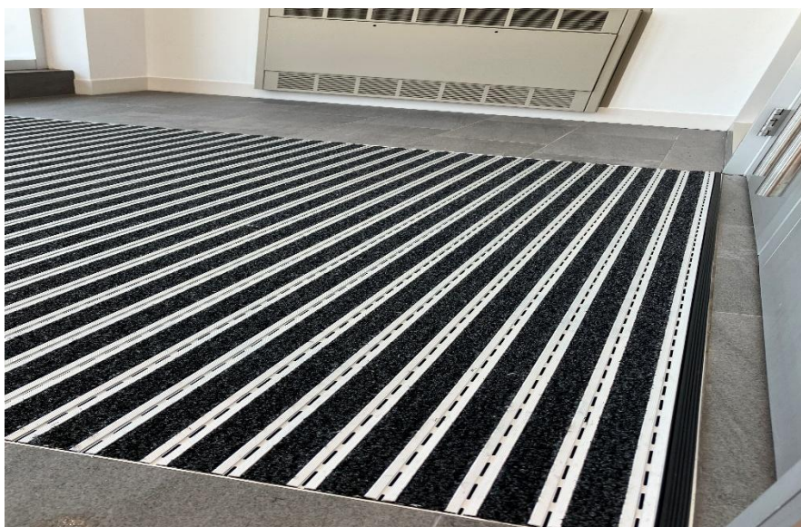
Aluminum entrance mat at an auto dealership with a black-grey blend to camouflage dirt and debris.
