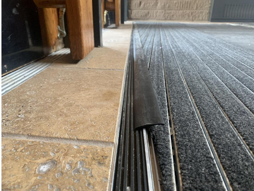
Close up view of the rails and the angled cuts for the entrance mat.
